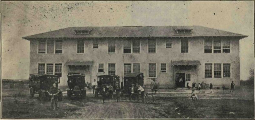
A. & M. Consolidated Building
